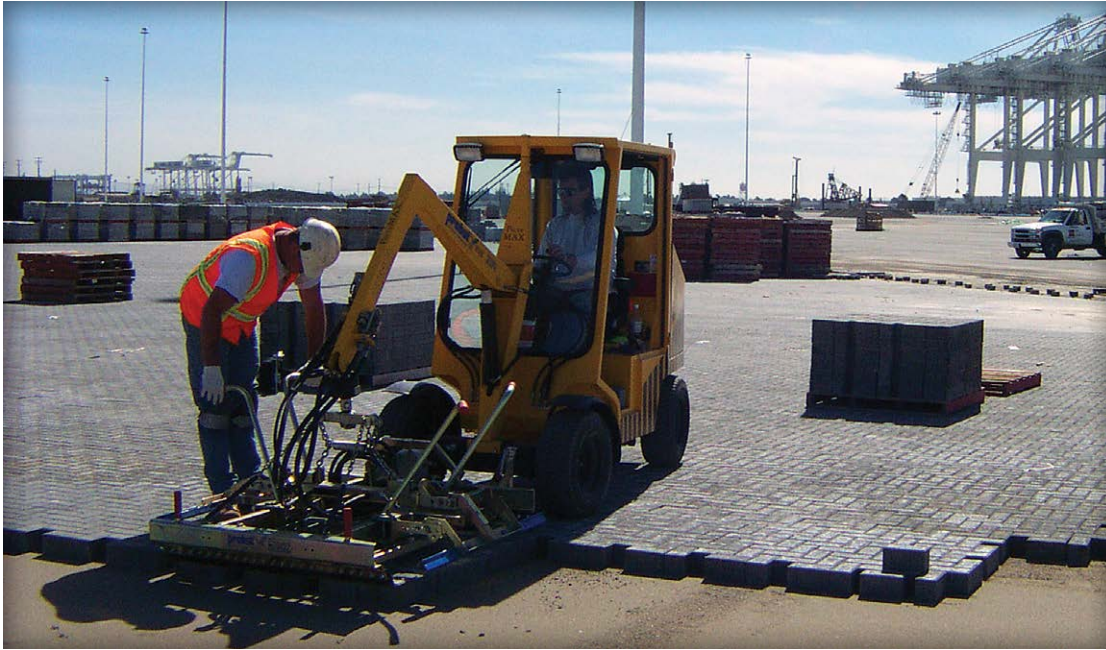
Figure 8. Mechanical installation equipment places concrete pavers rapidly.
