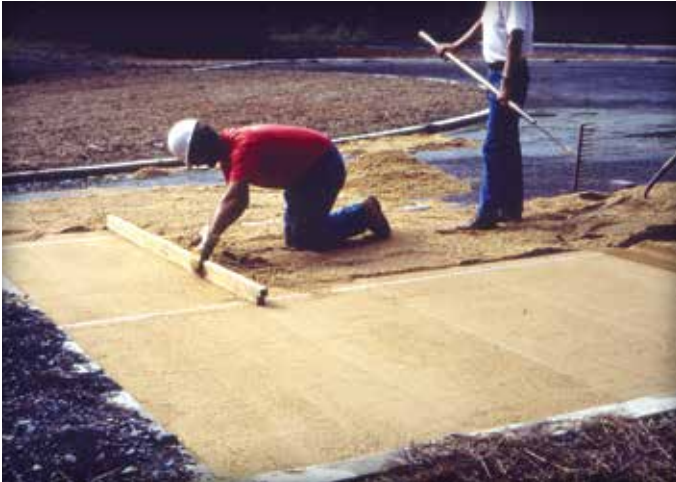
Figure 6a & 6b. Screeding the bedding sand.
